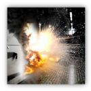
Fig. 1: Typical Arc Flash in Control Room
